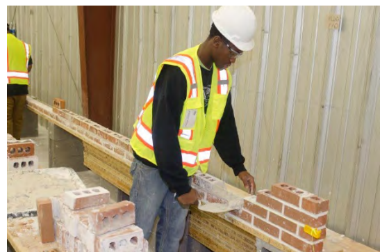
Student laying bricks for a wall in a Simulated Workplace in Alabama.
